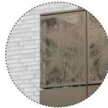
Perforated wind screen required on some balconies - refer to GA Plans & Elevations
